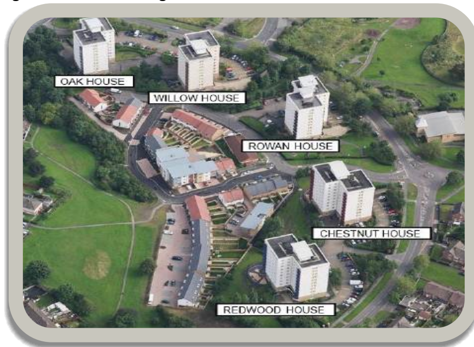
Figure 3 – Social housing blocks connected to the Rowan Heat Network
